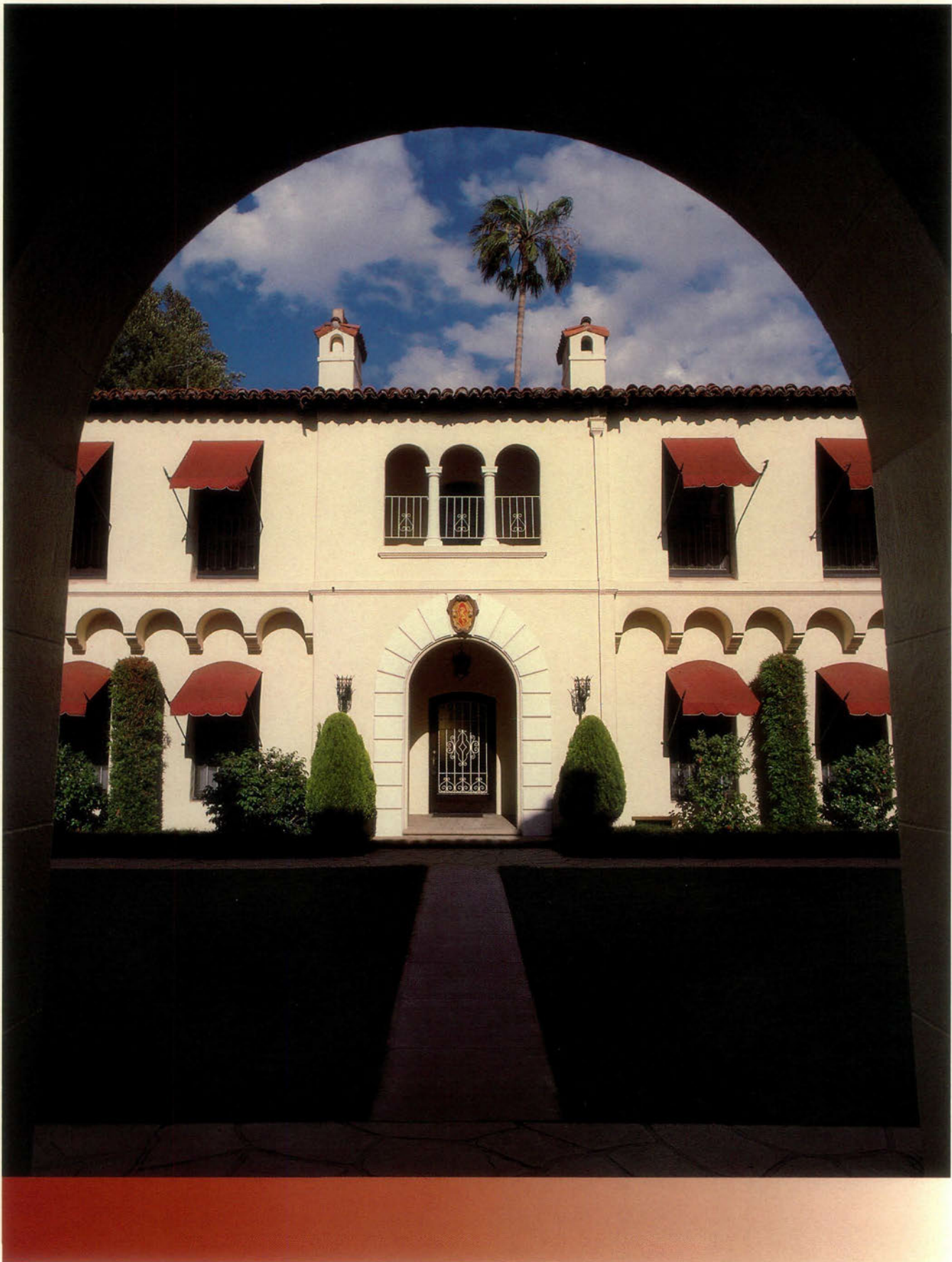
Within Grove Villa East are four apartments that have been converted to accommodate 12 students each. Grove Villa East is a residence for 48 men. A twin structure, Grove Villa West, is home for 48 women. This view is from the arched doorway of the women's residence looking toward Grove Villa East.
